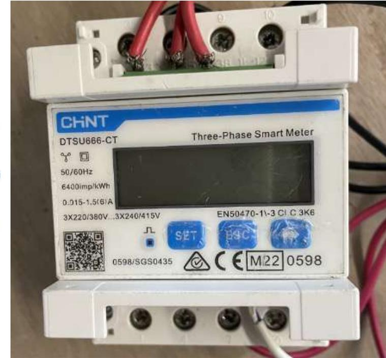
1. The meter should be CHINT DTSU666-CT, and the Eastron meter series currently does not support C&I inverters and Datahub.
