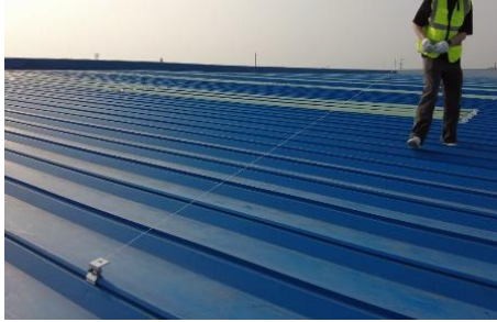
① Mark the Roof
