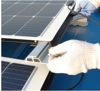
④ Slide the mounts into the brackets and screw the mount onto the base.
