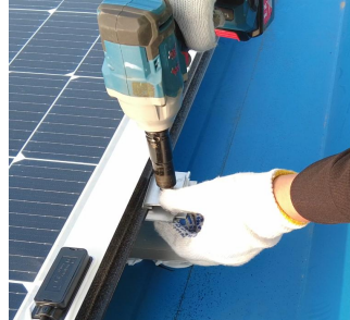
④ Slide the mounts into the brackets and screw the mount onto the base.
