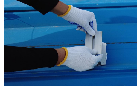
③ Glue the base to the roof
