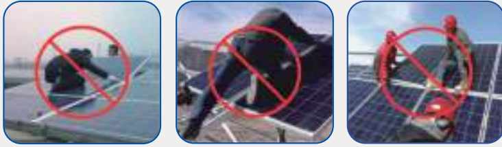
Don't step, stand or sit on modules while installing or cleaning.
