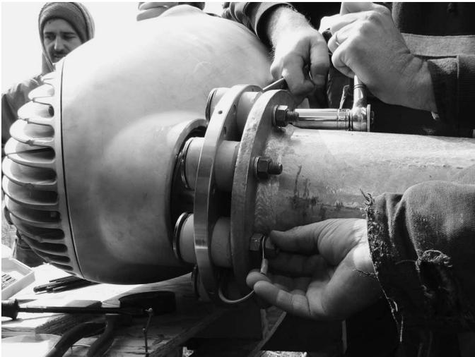
Fig. 10 Grounding turbine to tower
