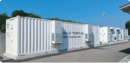
Switzerland Baden 2MW/2.17MWh Li-ion Battery Energy Storage System
